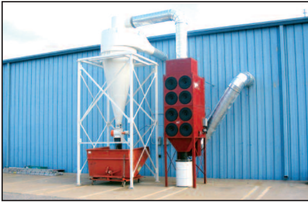
RP8 ducted to wood finishing operation
